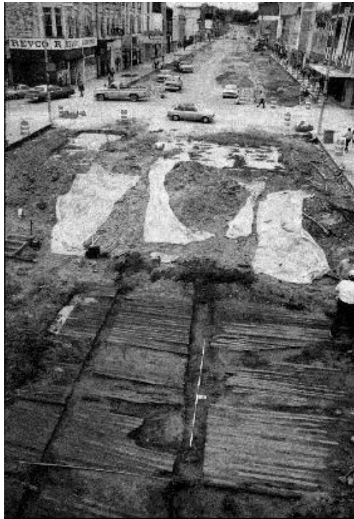
Excavation in downtown Fayetteville, North Carolina, during the 1980s, of the Fayetteville and Western Plank Road that was originally built in 1849.
